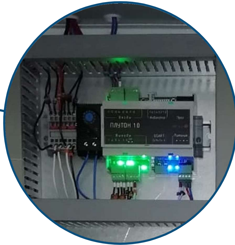
Ventilation control system cabinet based on PLC PLUTON for industrial painting station
