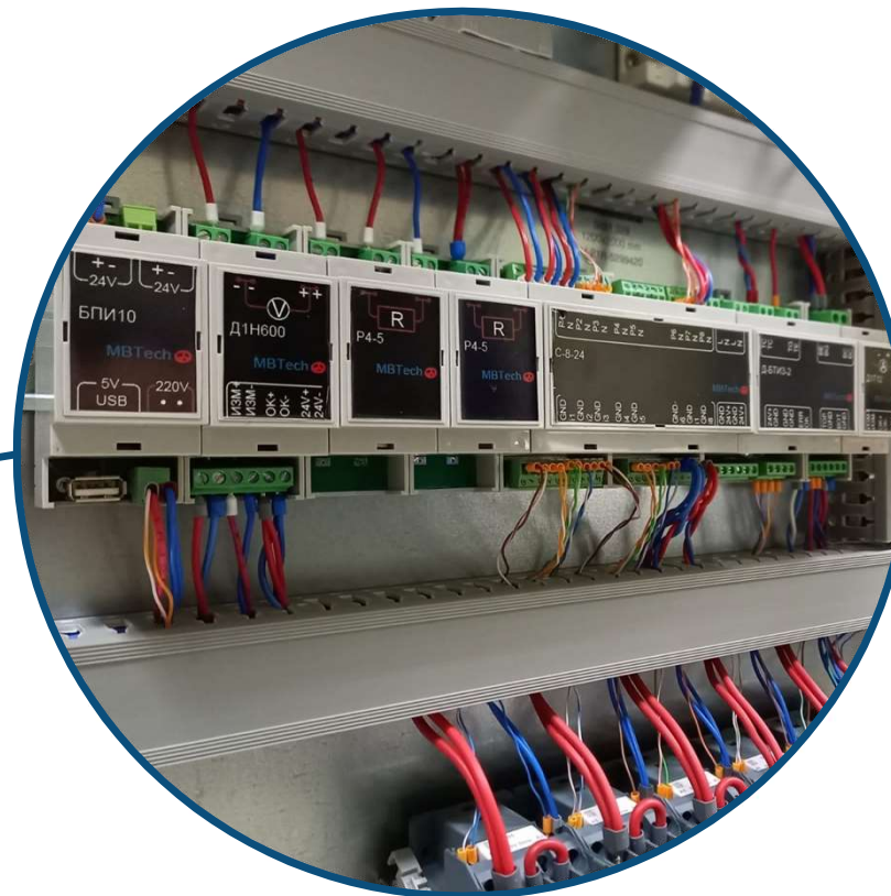
Control cabinet for road anti-icing automation system in Moscow based on PLC MAKON
