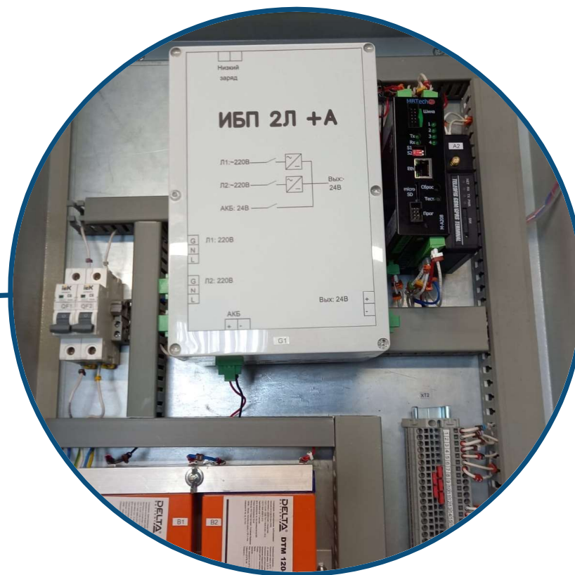
Monitoring system cabinet based on PLC MAKON
